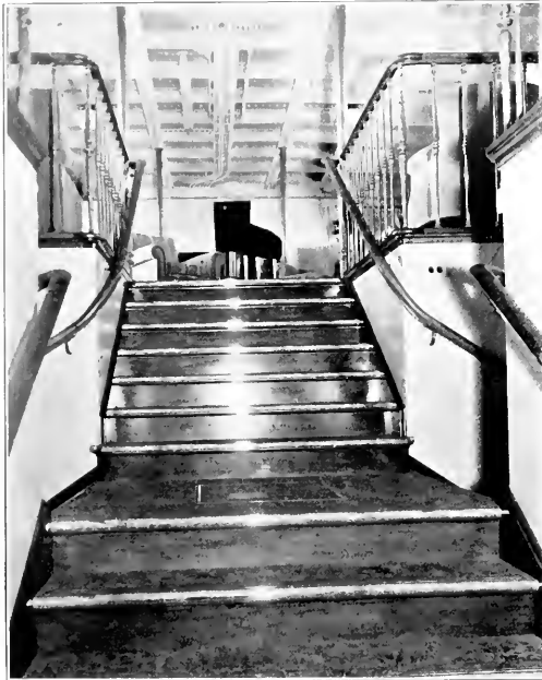
Three-way staircase on the Velero III. Note neat appearance of exposed wiring and deck beams.
